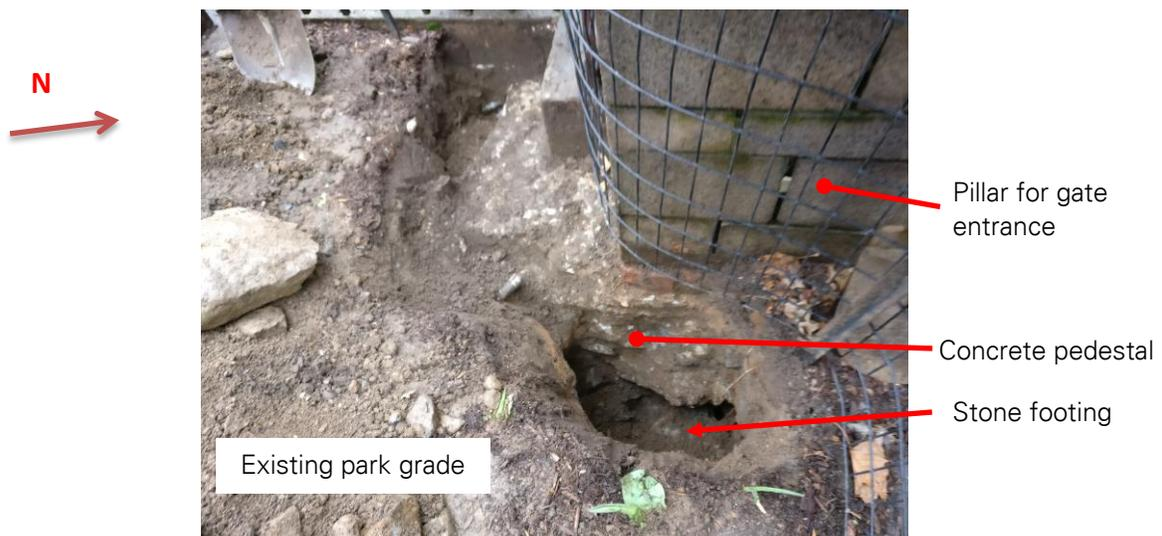
Photo No. 37: LTP-5, View of the fence foundation (View: West)
