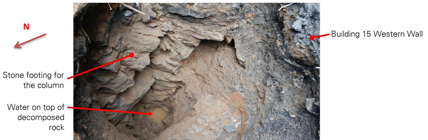
Photo No. 15: TP-5, Close-Up View of foundation footings (View: East)
