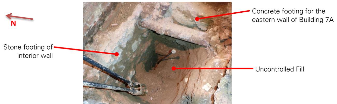
Photo No. 12: TP-4, General view of the test pit (View: East)
