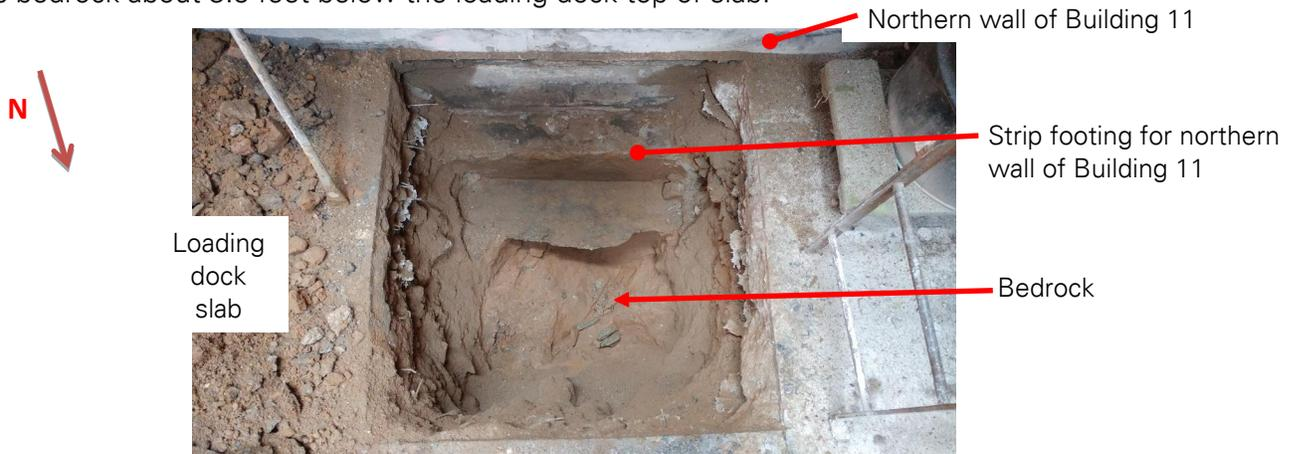
Photo No. 25: TP-11, General view of the test pit (View: South)
