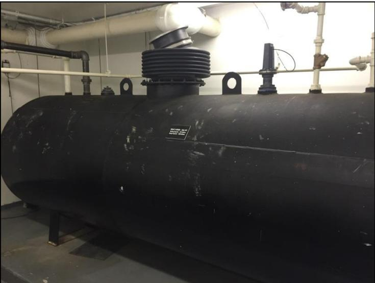
**Photograph 11.** 1,080-gallon diesel AST in Section 16.
