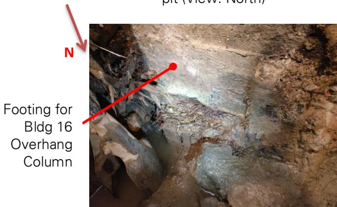
Photo No. 4: TP-1A, View of the Building 16 overhang column footing (View: Southwest)
