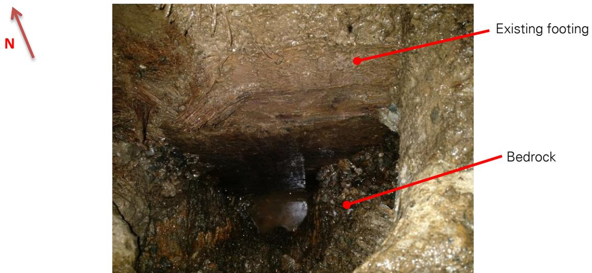
Photo No. 21: TP-8, View of foundation (View: Northeast)
