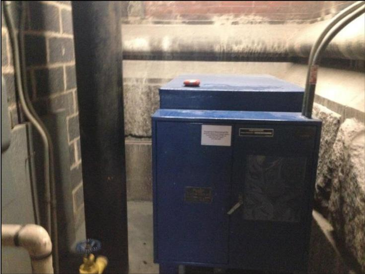
**Photograph 9.** Elevator mechanical room with hydraulic oil tank in Section 15.
