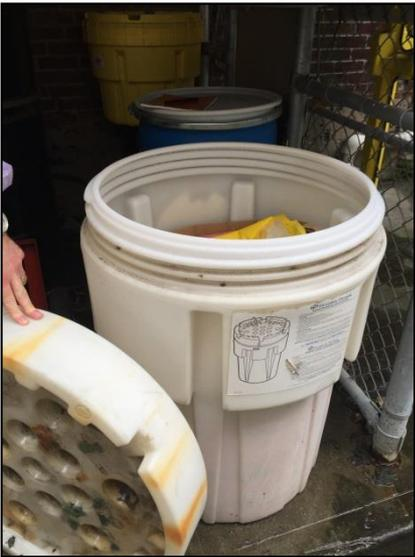
**Photograph 17.** Spill kit stored in the exterior yard chemical storage area.
