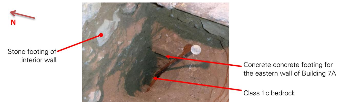
Photo No. 13: TP-4, View of foundation footings (View: East)
