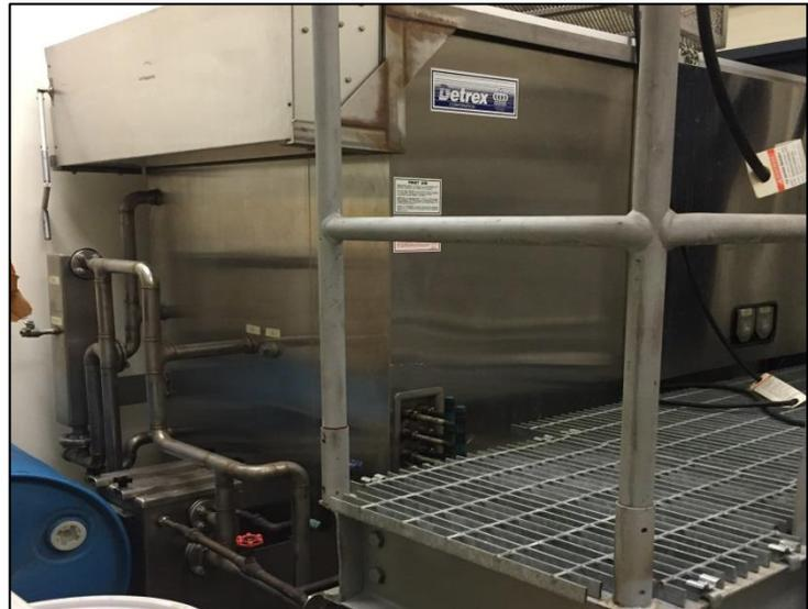
**Photograph 12.** Parts washer associated with degreasing operations and a decommissioned 250-gallon parts washer tank of trichloroethylene (TCE) in Section 17.
