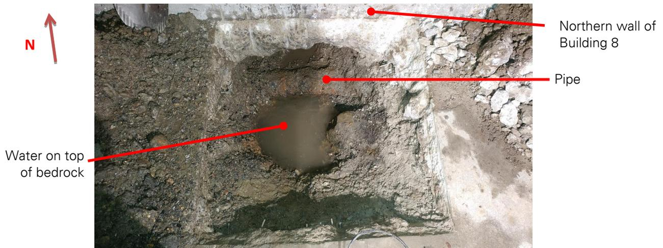
Photo No. 22: TP-9, General view of the test pit (View: North)
