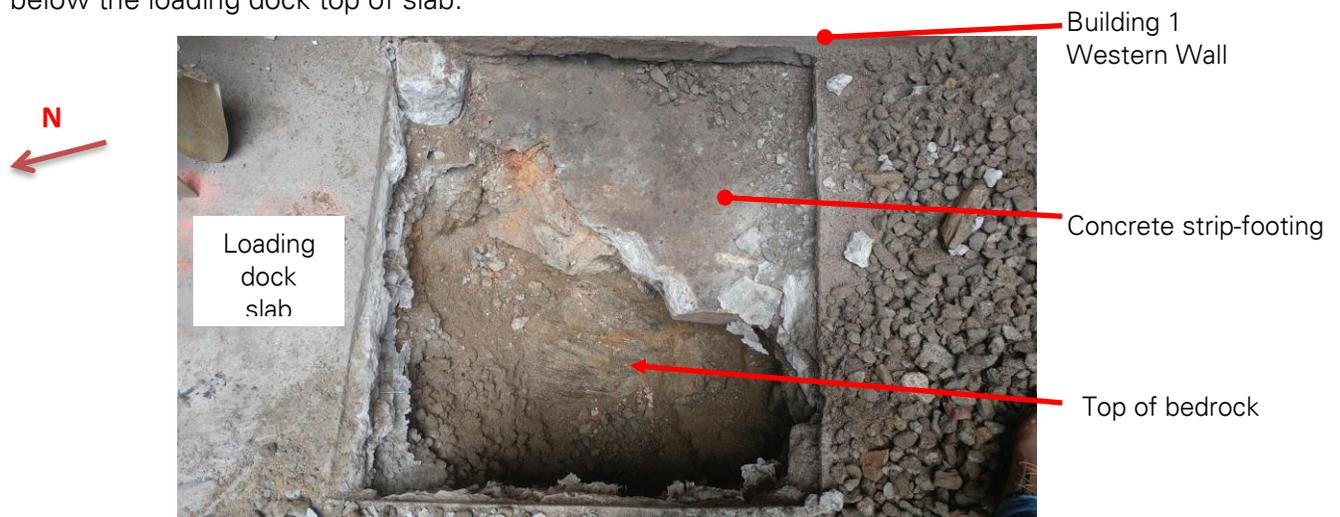
Photo No. 18: TP-7, General view of the test pit (View: East)
