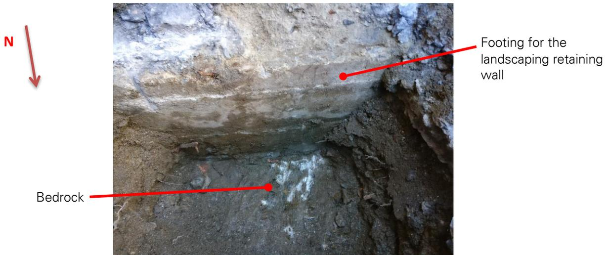
Photo No. 29: TP-13, View of foundation footing (View: South)
