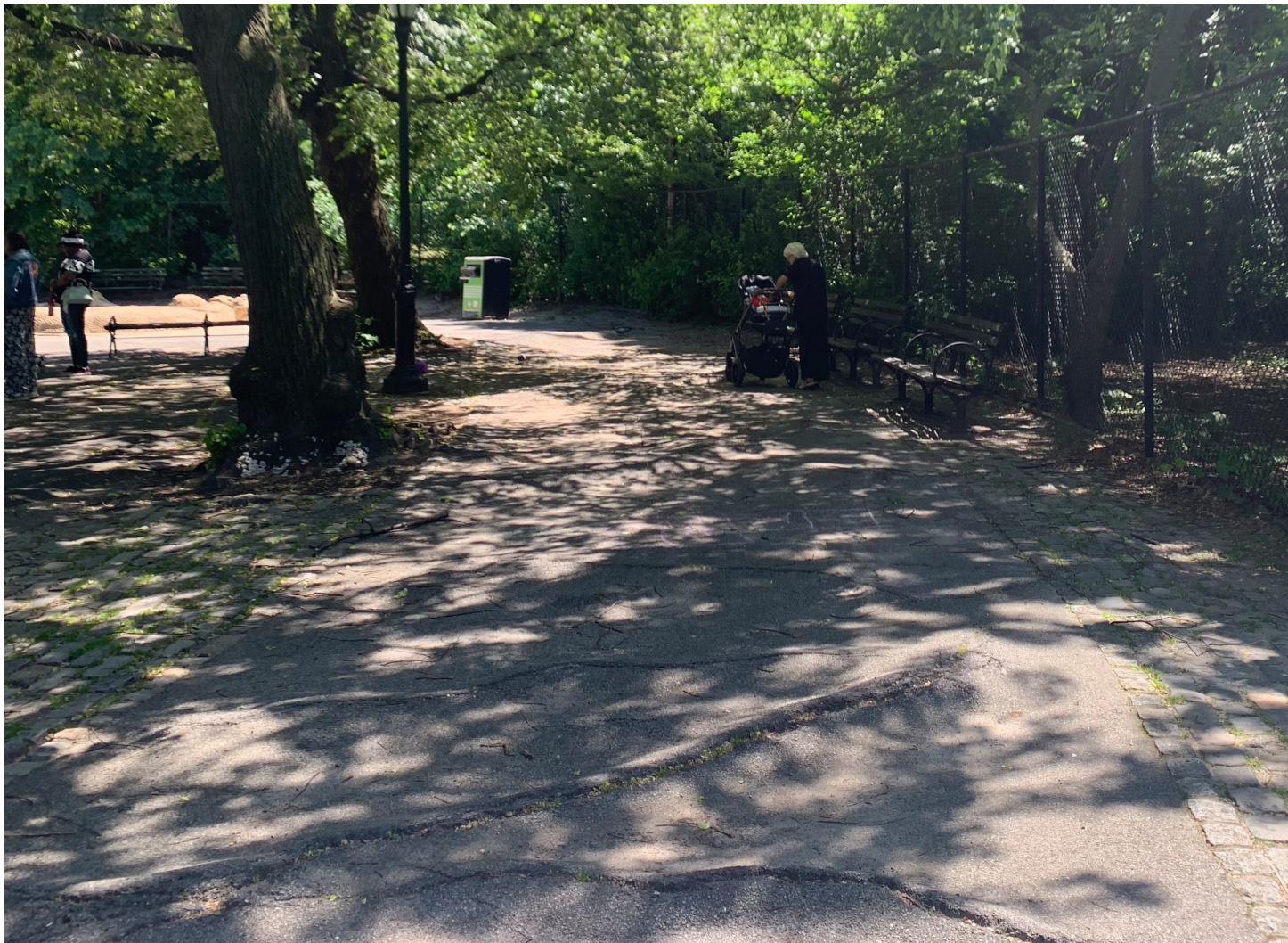
11 - Cracked & heaving asphalt pavement due to tree roots
